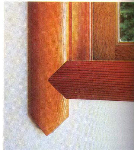
Windows and door are cased with rounded trim stock milled from select 2x4s (left). Half-lap bird's-mouth joints at trim intersections (detail above) are used throughout the house, and were milled in place with routers.
