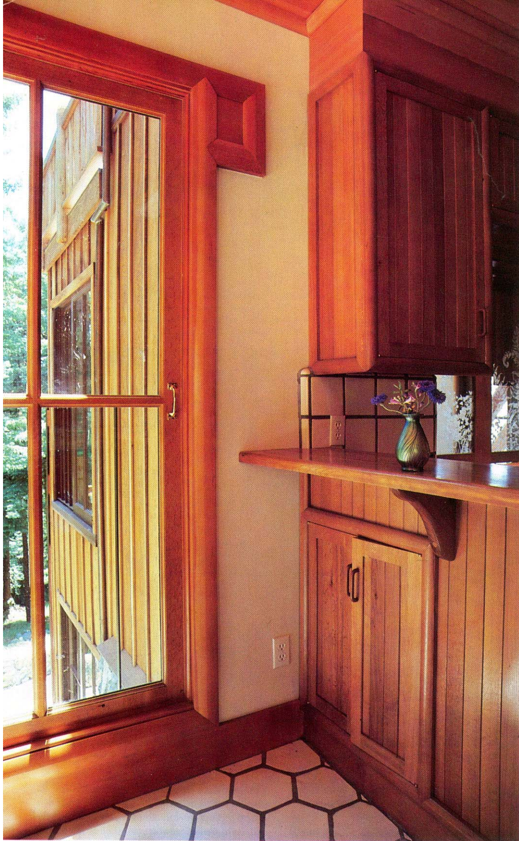
Windows and door are cased with rounded trim stock milled from select 2x4s (left). Half-lap bird's-mouth joints at trim intersections (detail above) are used throughout the house, and were milled in place with routers.
