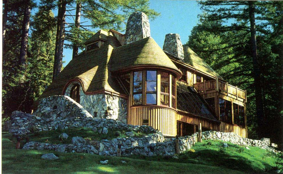
Clarke Shultes' design for a house in a redwood forest pays homage to the trees in form and color. The steep roofs with rounded hips echo the silhouettes of the trees in the background, and the cedar shingles tinted green mimic the surrounding foliage.
